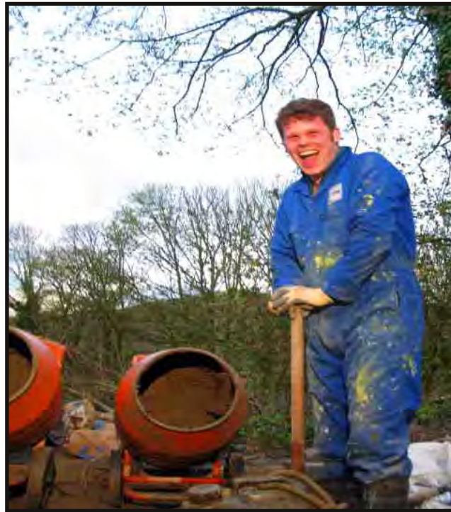
Jim Thompson mixing concrete on the surface Photo: Rob Eavis
