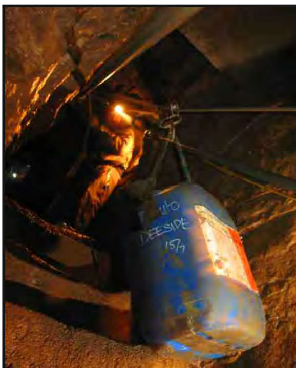
Kibble full of concrete Photo: Rob Eavis
